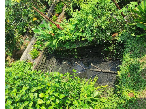
STP – Treated water is used for vegetation, Govardhan Eco Village
